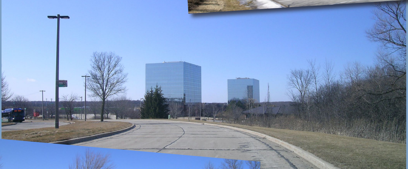
Today's neighborhood-Looking west at the twin 12-story office buildings, One Park Plaza and Two Park Plaza, on W. Lake Park Dr.
