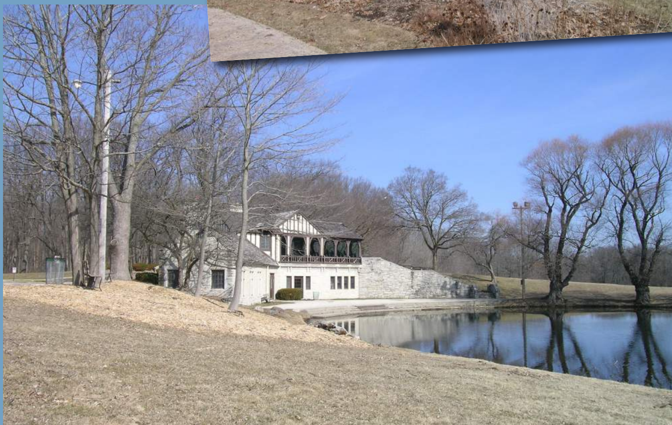
Today's neighborhood-Park boathouse pavilion
