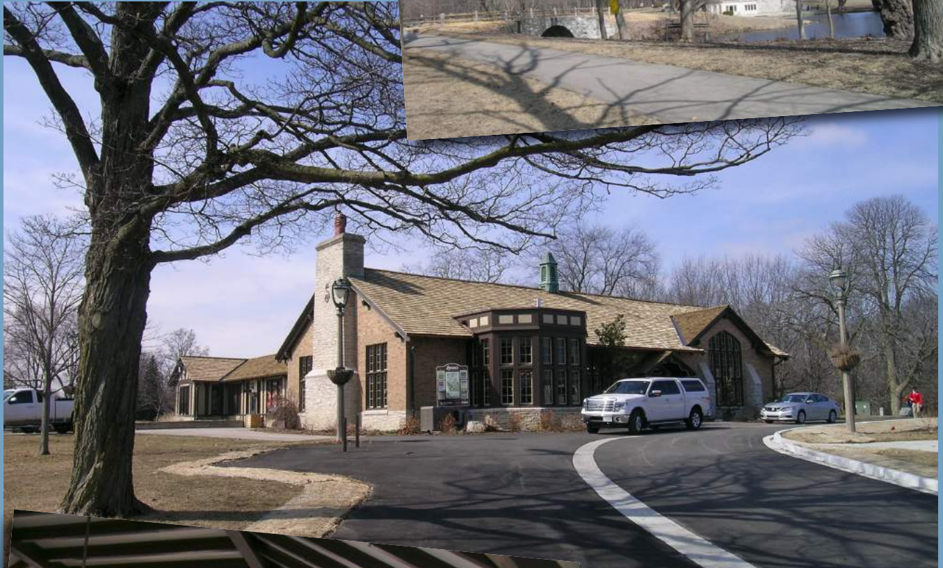
Today's neighborhood- Golf Course clubhouse exterior
