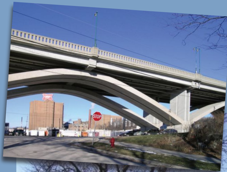
Today's neighborhood- Wisconsin Avenue Viaduct at 40th & Bluemound Rd.
