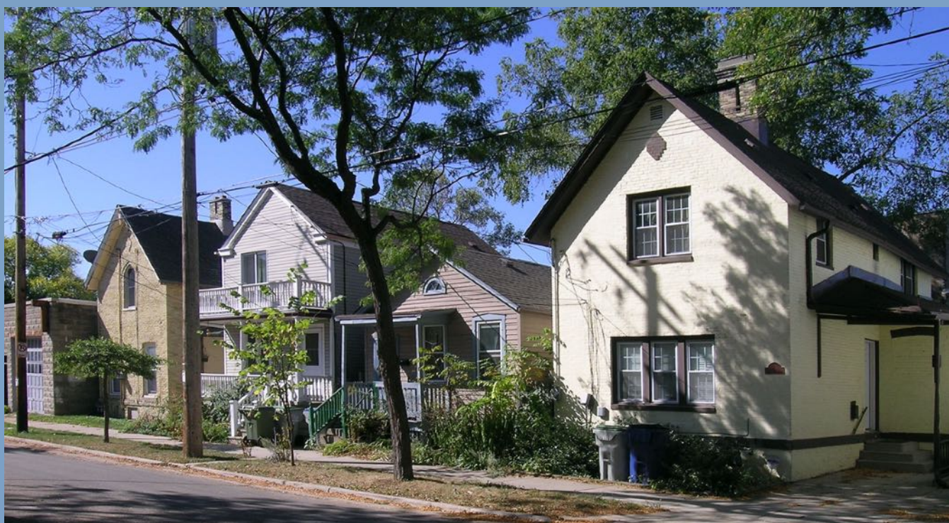
Today's neighborhood-Houses on E. Land Pl. & N. Marshall St.
